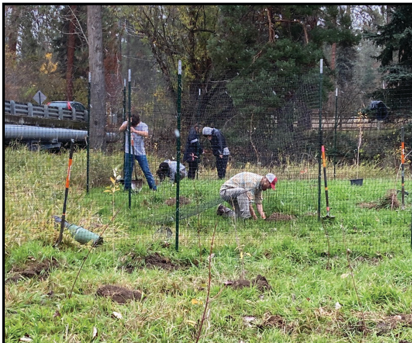
Students from On Track Academy helping with restoration work.
