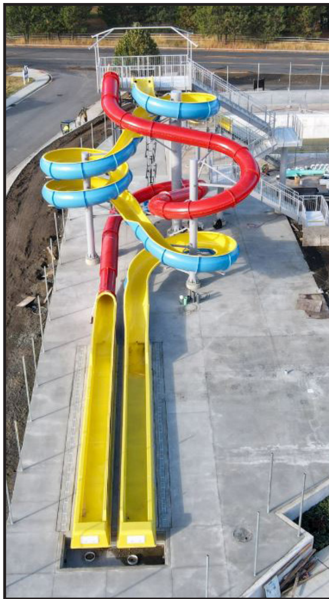
New water slide at Northside Family Aquatic Facility.
