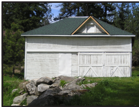
April 2011 picture. Windows to be added, siding repaired, and painting remaining.
