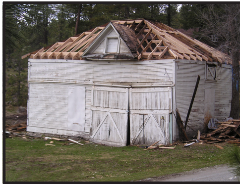
The barn in Spring 2011 undergoing repair. Because of wind and rain damage, many of the rafters needed replacing.
