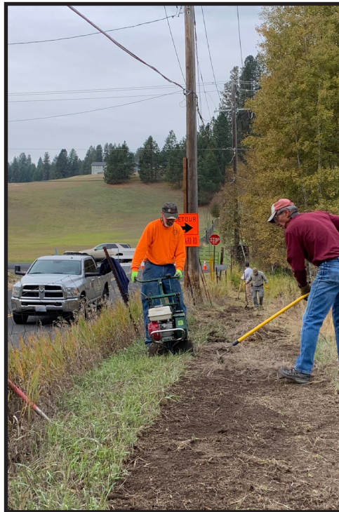
- Kirk With Sod Cutter, Dave Smoothing Out the Trail Bed -
